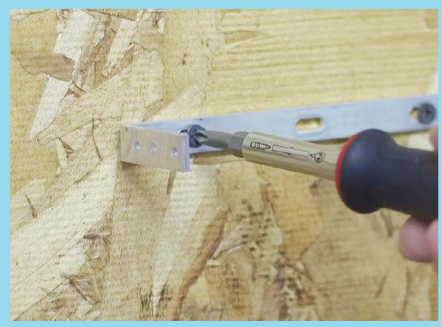
Attach the bracket to the wall.
