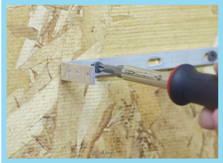
Attach the bracket to the wall.
